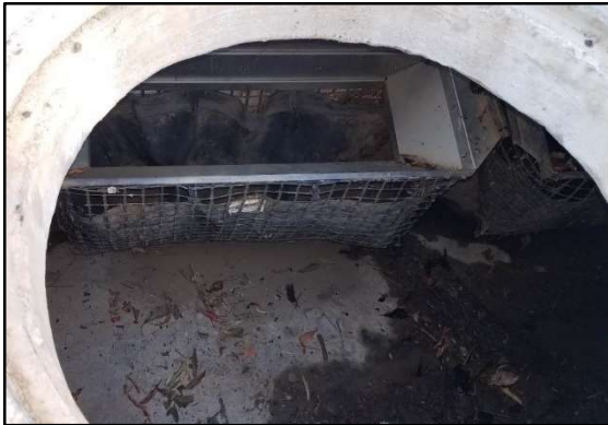
Figure 3. Installed FloGard® CIB - view from manhole.
