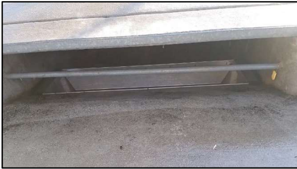
Figure 1. Installed FloGard® CIB – empty (view from curb).
