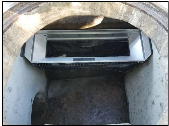
Figure 4. Installed FloGard® CIB – bottom of catch basin.
