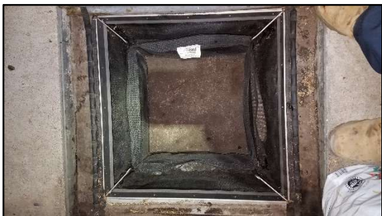
Figure 5. Installed FloGard® GIB – view to bottom.
