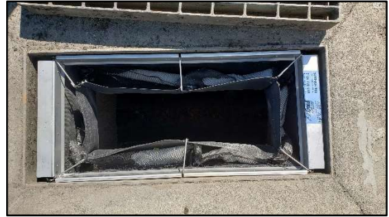
Figure 2. Installed FloGard® GIB without grate.
