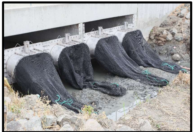
Figure 12. Completed installation of NetTech.
