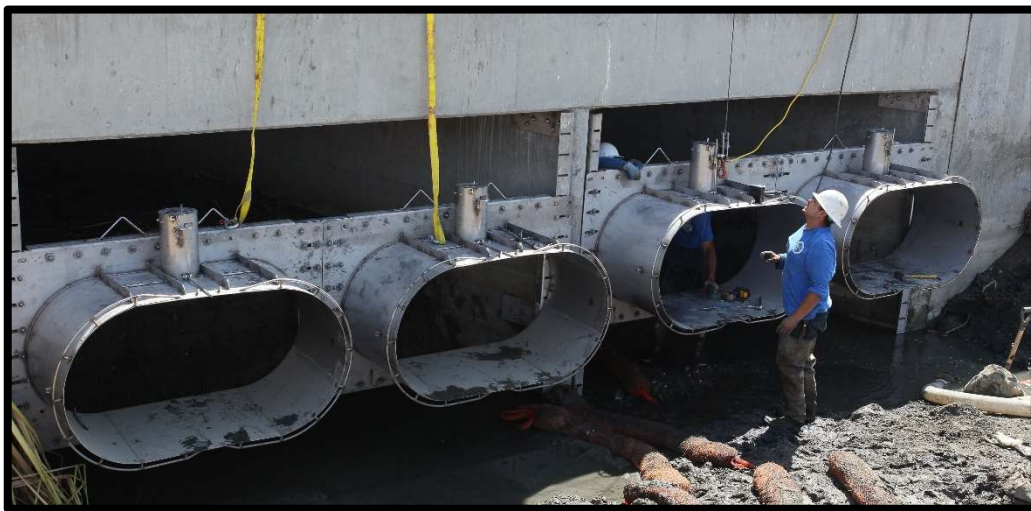
Figure 10. Installation of NetTech mounting brackets.
