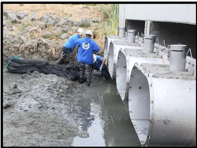
Figure 11. Installation of trash capture netting.
