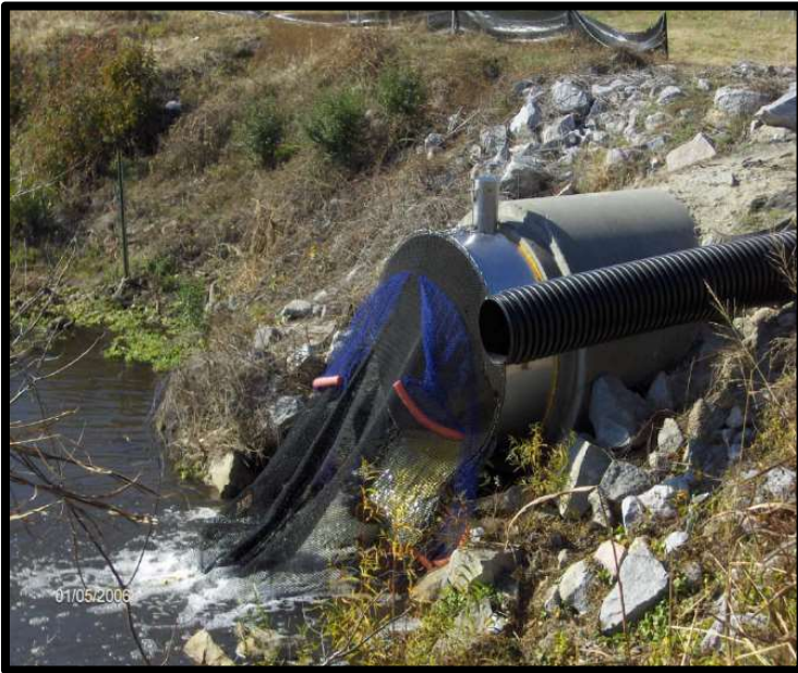
Figure 1. 72" RCP at continuous flow installation.
