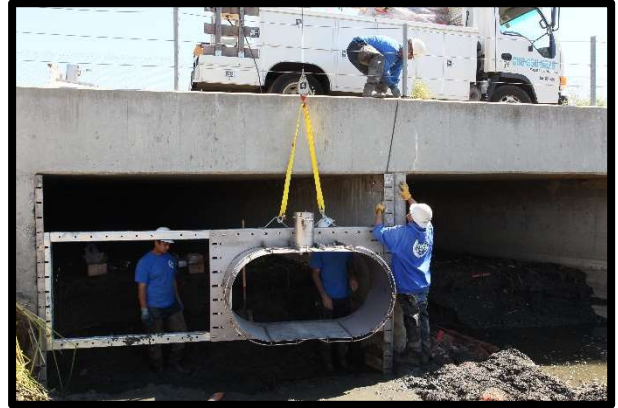
Figure 9. Installation and maintenance access from road.
