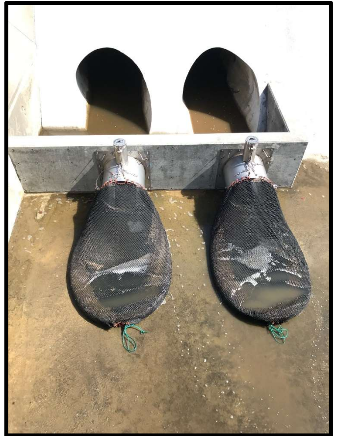
Figure 5. Installed NetTech at approximately 50% capacity.
