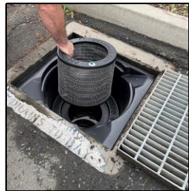
TR2424 Removing Cartridge
