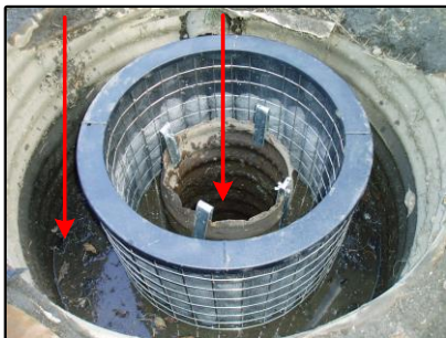
Area Drain Filter (ADF) shown in a trench drain with a vertical exit pipe.
