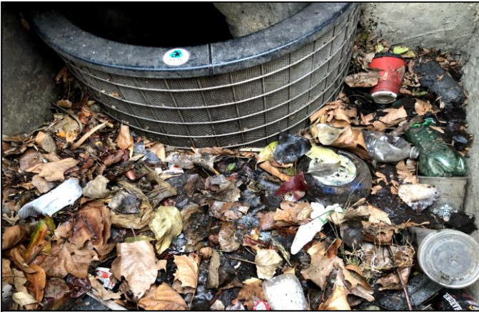
Test Unit T3: TR24(16)-CPS @ 40% Capacity 3 Months after installation – 60% Organic 40% Trash
