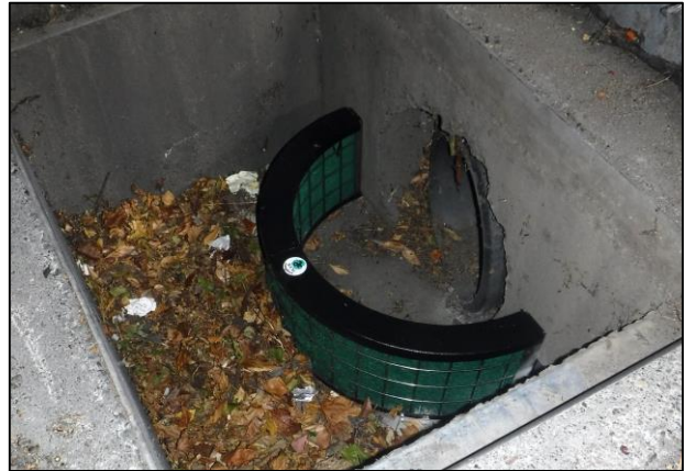
Standard REM CPS device installation (No deflector)
