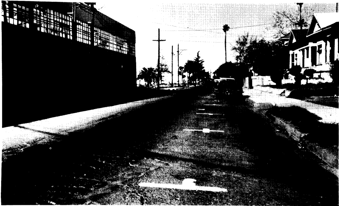
Figure C-7. Downtown - poor asphalt test area.
