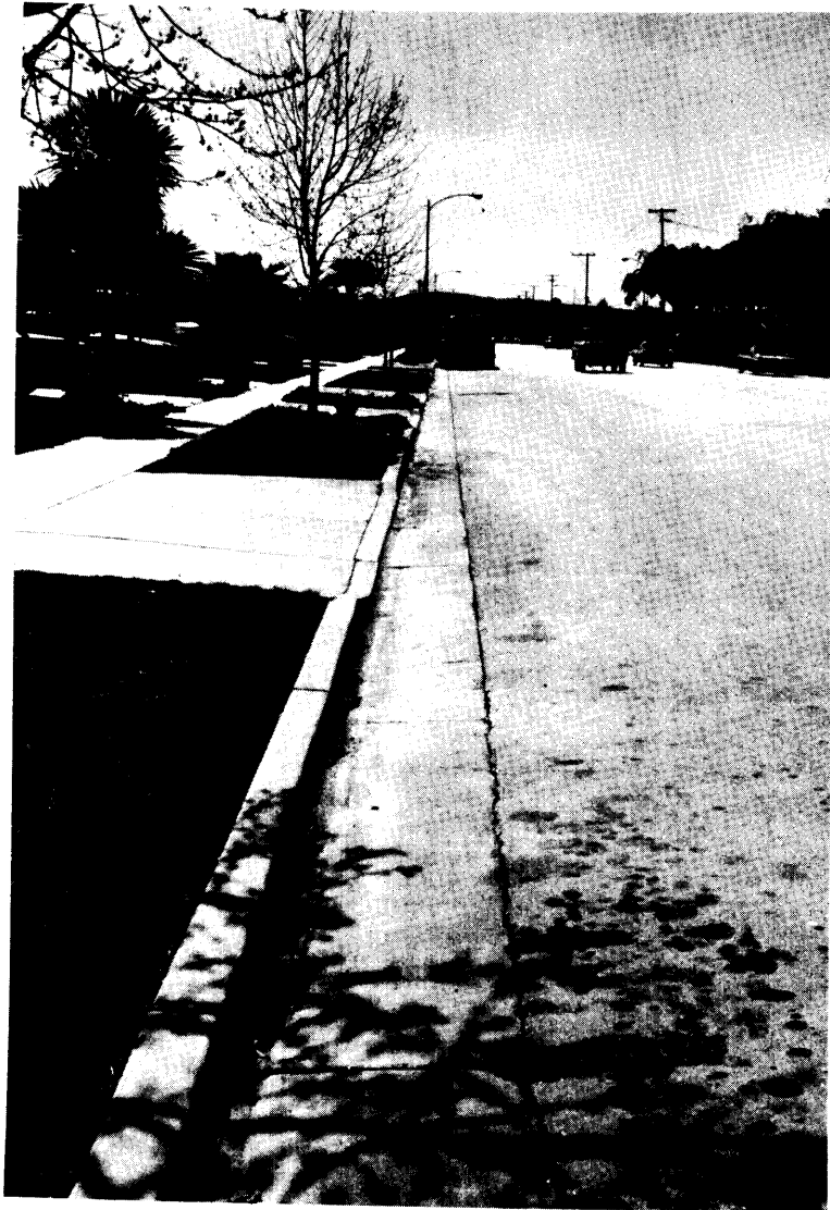
Figure C-10. Tropicana - good asphalt test area.
