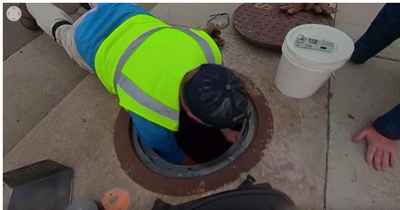
Image 11 - Attaching the final suspender to the rear/north side of the filter hanger after installation
