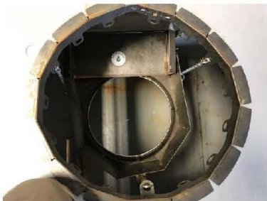
Image 7 - top view through manhole opening of CIF with Mundus Bag® removed showing the bottom of catch basin
