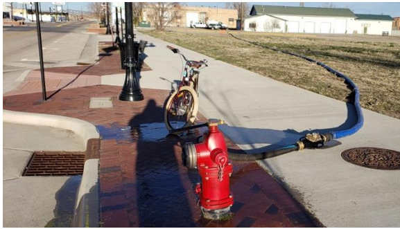
Image 14 - Adjustable hydrant meter water source - up to 350 gpm
