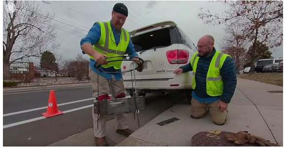
Image 10 - Assembling optional MFH, filter hanger and suspenders prior to installation in catch basin
