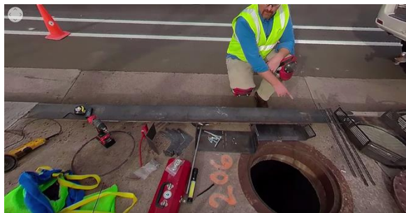
Image 3 - Pre-installation view showing gutter channel
