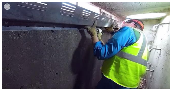
Image 5 - Marking initial anchor bolt position prior to drilling
