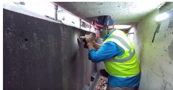
Image 6 - Drilling initial anchor bolt for gutter channel
