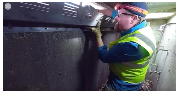
Image 4 - Determining proper placement of the gutter channel
