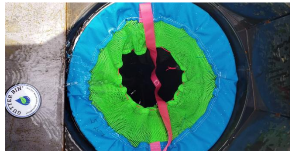
Image 17 - Overhead view of TDS-MB installed in test CIF
