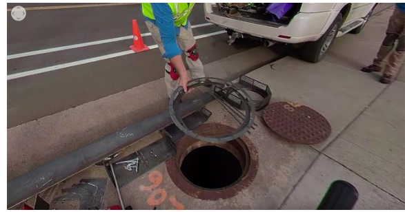
Image 2 - Pre-installation view showing optional adjustable MFH
