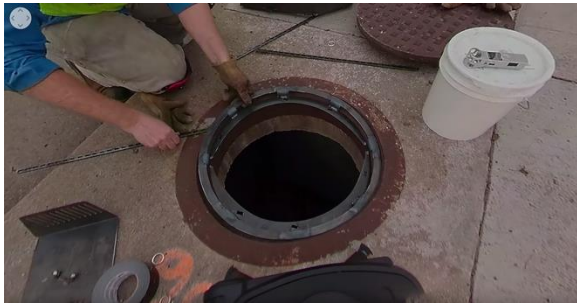
Image 9 – Test fitting optional adjustable MFH and determining ideal distance from which to suspend the filter hanger
