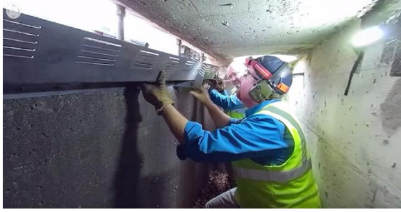
Image 7 - Installation of the gutter channel using gussets
