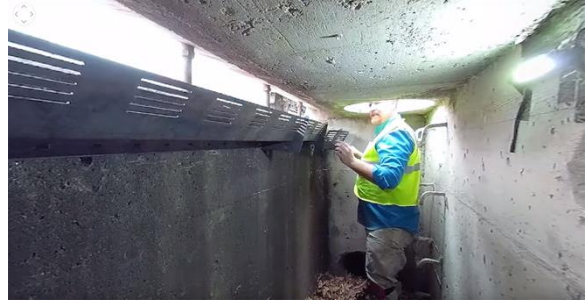
Image 8 - Installation of interface funnel
