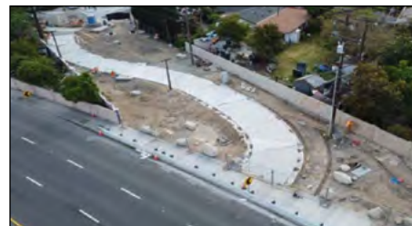
King Street Project's pervious pavement bike path during construction.
