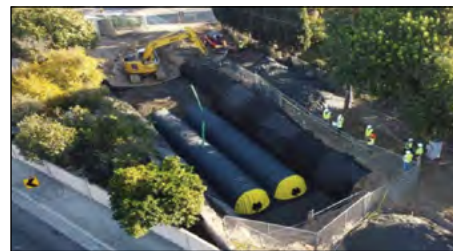
Aerial photo of subsurface infiltration system construction at King Street.
