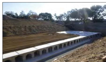
Backfill of the Subsurface Storage System.
